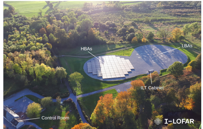
Fig. 1. Irish Low-Frequency Array station IE613 (I-LOFAR) at Birr Castle, County Offaly. Coaxial cables are used to transport data from the Low Band Antennas (LBAs) and High Band Antennas (HBAs) to the ILT Cabinet (centre right), where it is amplified, filtered, and digitalised. Data is sent in international mode at a speed of \sim 3.2 Gbps to Groningen, Netherlands. In the I-LOFAR Control Room, data is processed using REALTA in local mode (bottom left; Murphy et al. 2021).
